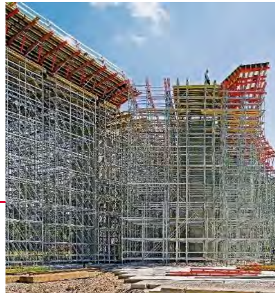
1998 PERI UP Scaffolding
