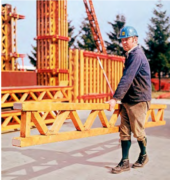
1969 T 70 Wooden Lattice Girder
