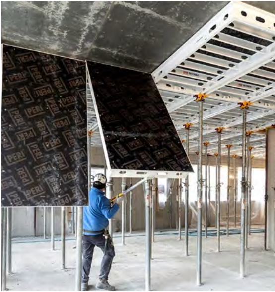
2019 SKYMAX Slab Formwork
